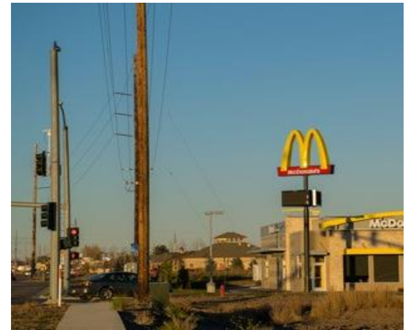
Rexburg: Moving Power Transmission Lines
